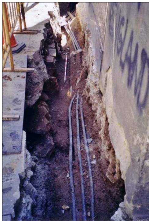
F4: Vista general del tram 3
